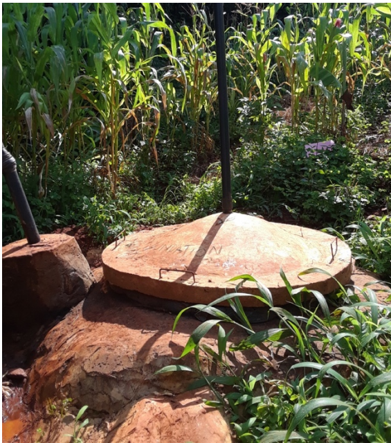
Figure 22 - Underground water basin and manual pump. Photo taken on my phone, June 2018. Point on map: WaLi Water Collection System
