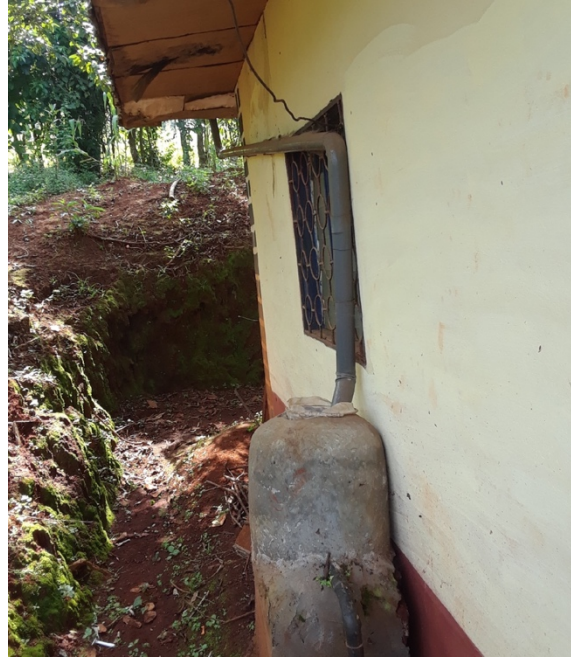
Figure 20 - Water from the gutters is then filtered and stored in a small container. Photo taken on my phone, June 2018. Point on map: WaLi Water Collection System
