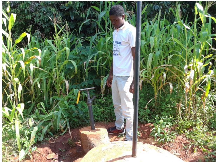
Figure 21 - WaLi Water Catchment System storage basin and manual pump ft., team member Judicaël. Source: photo taken on my phone
